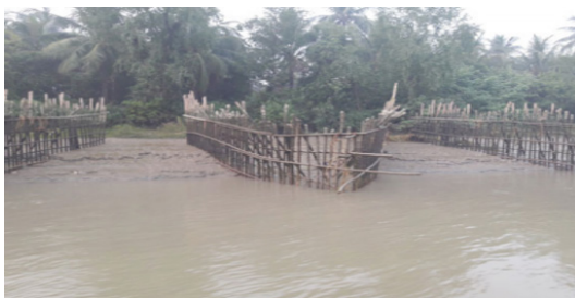
Fig. 8: Sediment deposition near the eroded bank within the bamboo bandals field 27
