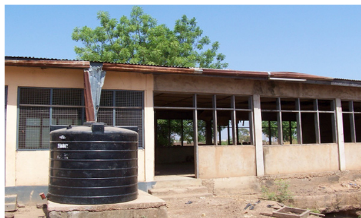
Fig. 8: RWH system in vocational school 10
