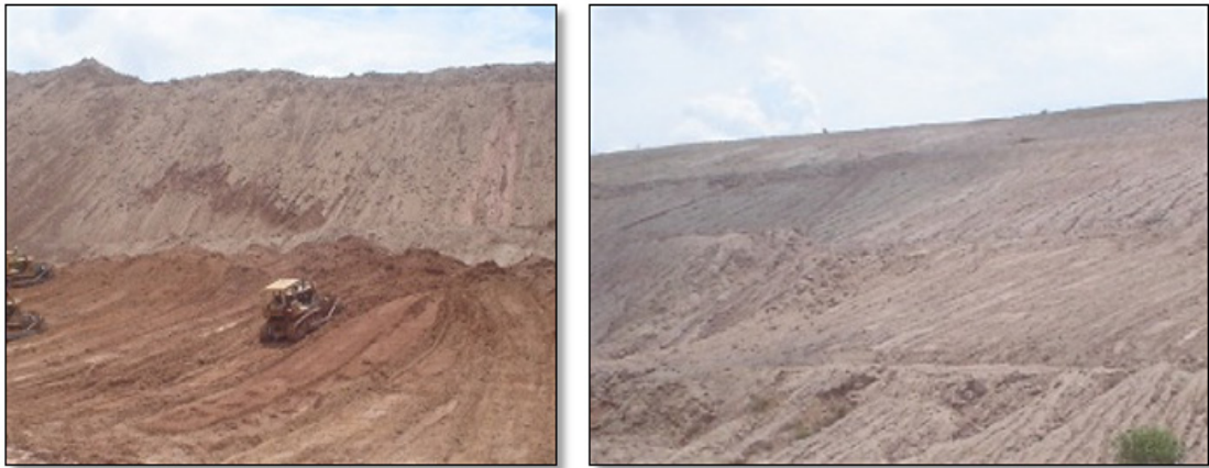
Fig. 3: Slope Stabilization with 5 benches
